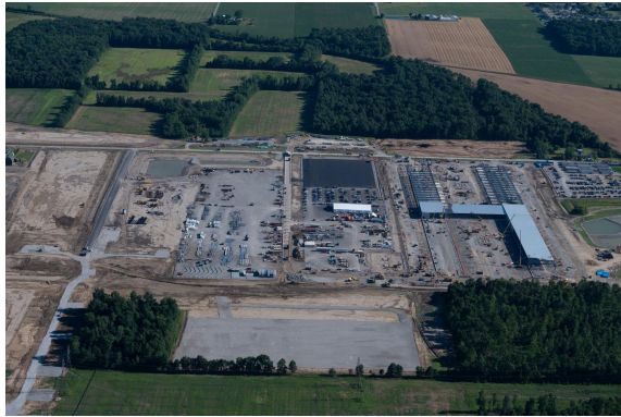
(B) Google Data Center
