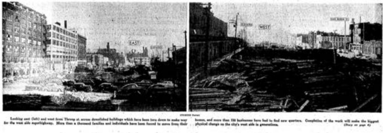
Figure A3: The construction of the Eisenhower Expressway, 1949
