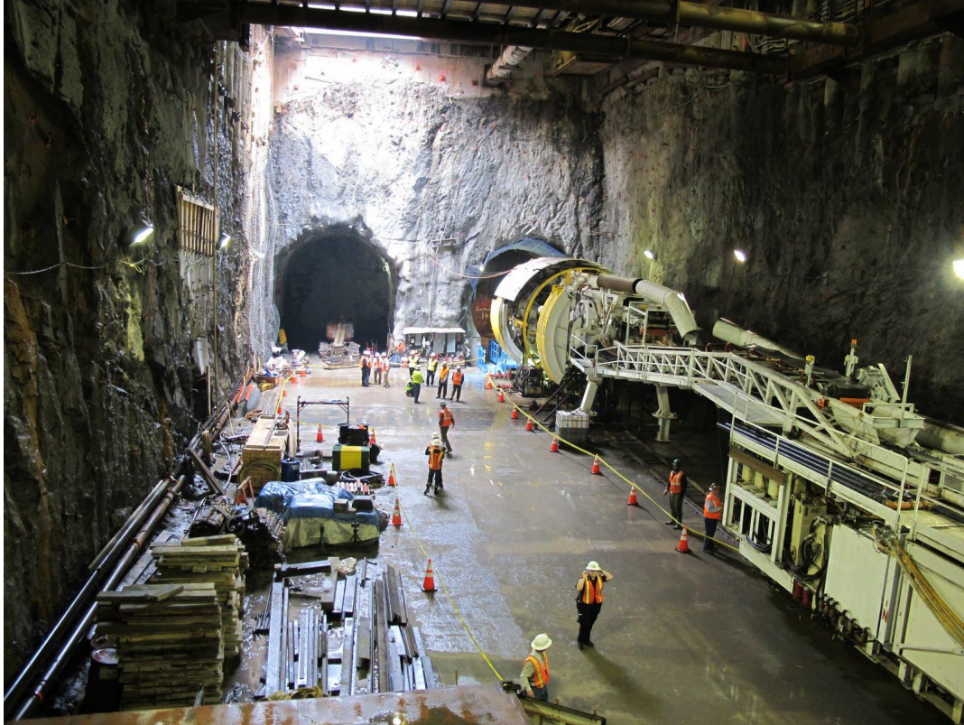
Second Avenue Subway TBM Launch Box
