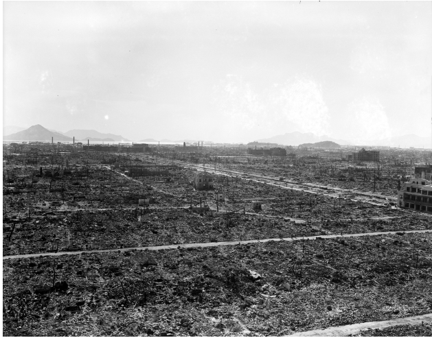
(a) Total Destruction Near the Epicenter
