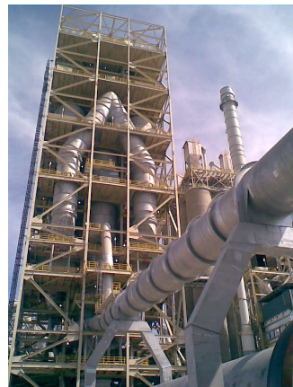
Cement Precalciner (Source: Cement Production)
