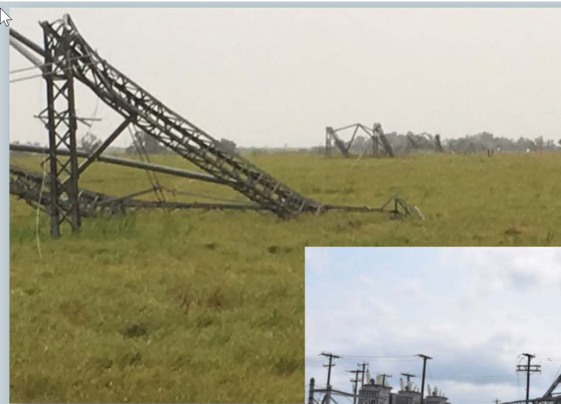
STP-to-Whitepoint 345-kV transmission structures
